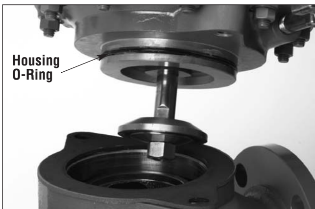
Fig. 26 Installing the Actuator on the Body.
